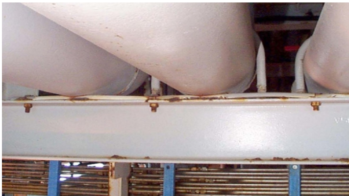
A CLOSER LOOK The same supports pictured above at 13 years. I-Rod is showing some signs of stress on the right pipe.
