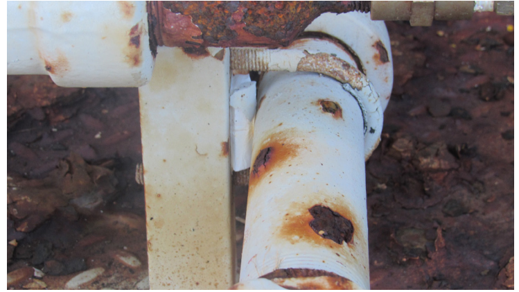
CLEAN CREVICE After 28 years the I-Rod shows no change long after the coating has failed.
