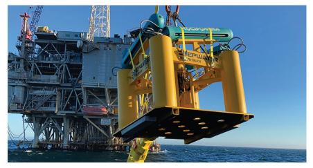
ONE DOWN, TWENTY TO GO Positioning a RetroBuoy™ for deployment in the largest offshore ICCP retrofit ever done in a single campaign.
