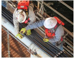
SAVING MONEY WHILE SAVING STRUCTURES Still-functional elements of the exising ICCP system were re-used to cut costs.
