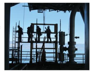
OUT OF HARM'S WAY Junction boxes were raised an extra 11 feet to prevent flooding in high seas.
