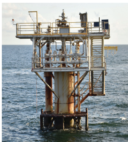
PLATFORM IN 66 FT. DEPTH Three 66' RetroLinks™ with 25' leaders were used.
