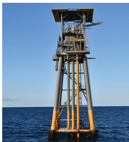
PLATFORM IN 150 FT. DEPTH 11 longer 150' RetroLinks™ with 25' leaders were used.
