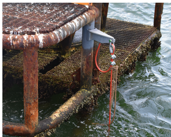
THE RETROLINKS™ WERE HUNG FROM WELDED-ON STAND-OFFS. At least two of the anodes on each string lie in the mud.
