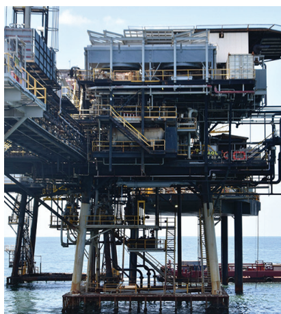
PLATFORM RISER WAS ELECTRICALLY ISOLATED A VampClamp™ now provides electrical continuity.
