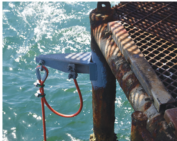
QUICK INSTALLATION IN 66 FEET OF SEAWATER RetroLinks™ are almost always installed from a small boat without divers.
