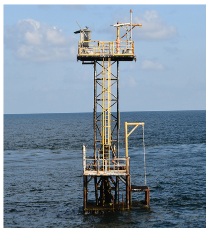
(ANOTHER) PLATFORM IN 66 FT. DEPTH Three 66' RetroLinks™ with 25' leaders were used.
