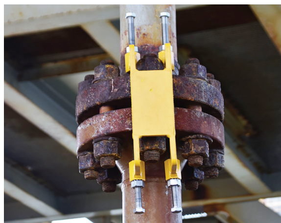
DEEPWATER'S VAMP CLAMP™ INSTALLED The Vamp Clamp™ ensures electrical continuity across insulated flanges..
