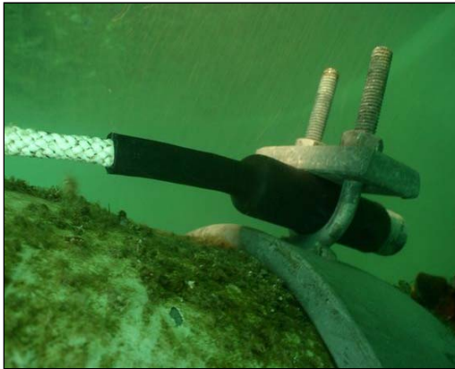
V-String reference electrode in situ on a retrofitted CP monitoring system.
