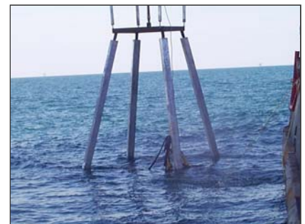
This illustration shows the Clamp installed by an ROV.
