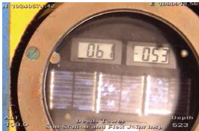
A first-generation SunStation as recorded by the inspecting ROV.
