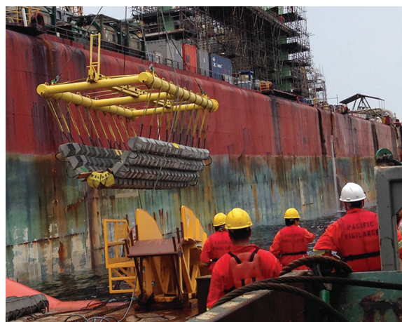
STAYING IN PLACE A concrete mat keeps the cable in place on the sea floor.
