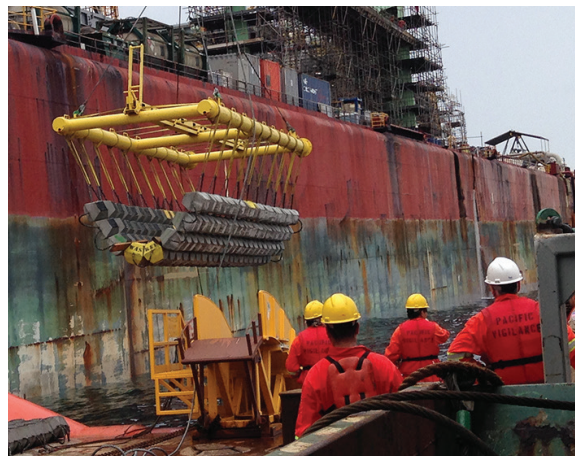
STAYING IN PLACE A concrete mat keeps the cable in place on the sea floor.
